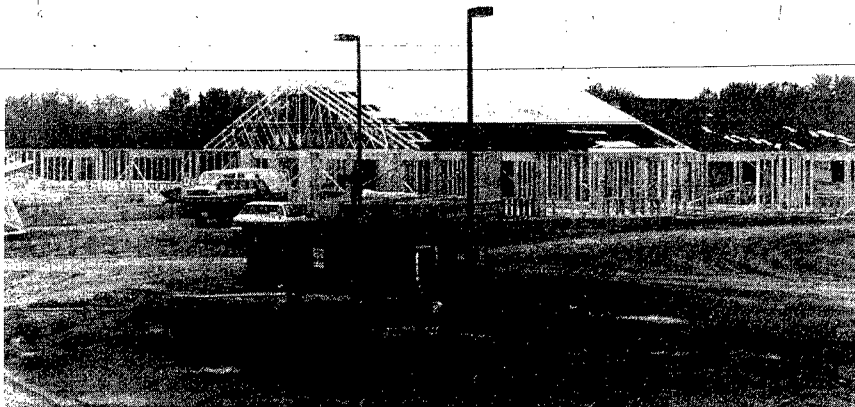
Construction is proceeding at a rapid pace on the new Wayne Care Centre project as contractors scramble to make up time lost to unprecedented weather delays.
